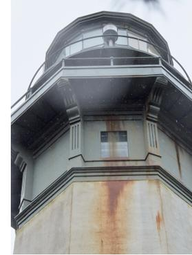
Metal corrosion / wall staining
