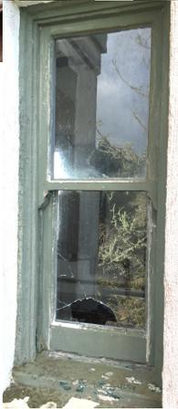
Deteriorated window sills / glazing
