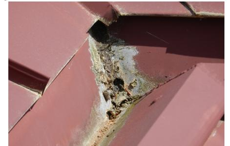
Hole in gutter / improper slope
