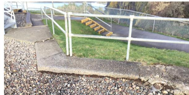
Sidewalk cracks and heaving
