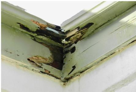
Deteriorated gutter & fascia
