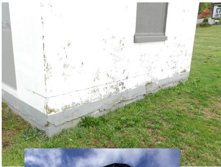
Stucco spalling / poor drainage away from building
