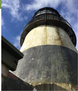
Wall staining and spalling stucco
