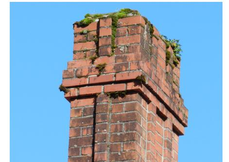
Organic matter on chimney/deteriorated brick
