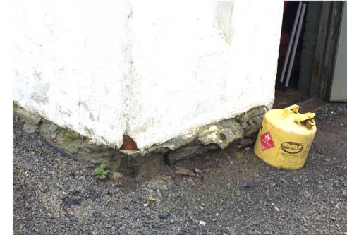
Deteriorated foundation / combustibles in building
