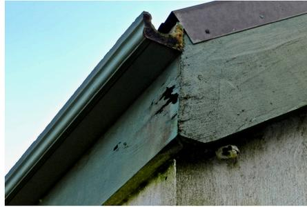
Missing gutter end cap / deteriorated fascia
