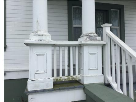
Columns, bases and railing deteriorated
