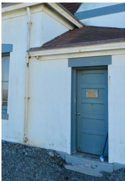
2 Downspout blocked or corroded
